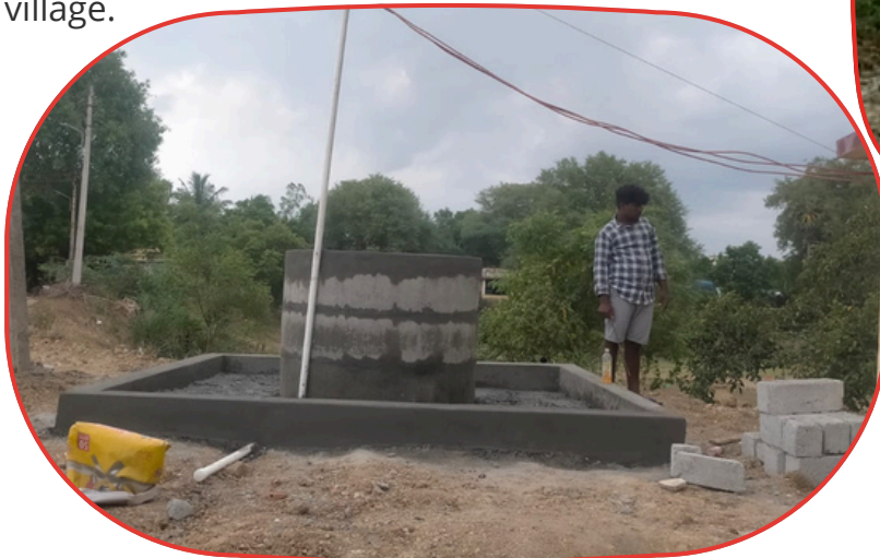
Stage 2: Motor Installation & Storage tank Basement Construction
